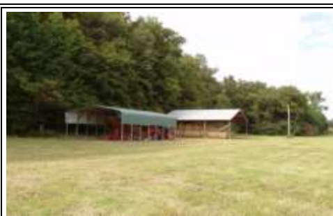
Equipment / Hay Shelter
