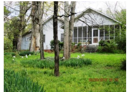
Front view of home
